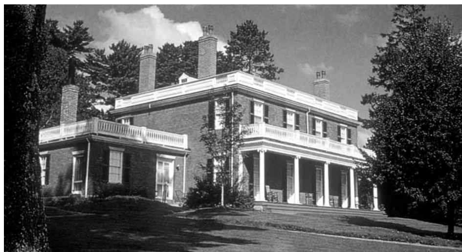
Front facade of the mansion.
